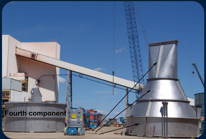
SNC-Lavalin Inc.: Saskatchewan, Canada Loadout/Blowback Dust Surge Bin – 2205 Stainless Material (4 Separate Components)
