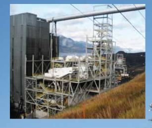
In 2011, we were contracted to detail and fabricate all the required structural steel for a new preparation plant and loadout facility. This included structural steel columns, beams, bracing, bins and plate work, miscellaneous steel, handrails, platforms, and grating, as well as a multi-coat paint system.
