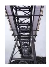
In 2011, we were contracted to detail and fabricate the Bloom Lake iron-ore-handling system for Cliffs Natural Resources in Quebec, Canada. The project consists of a 2-1/2-mile super elevated and horizontal curving overland conveying system with associated support bents, transfer towers, and iron ore storage building.
