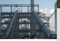
In 2008, we completed a limestone-handling system, which provides 24/7 service with a capacity of 3,400 tons per hour, for Southern Company's Plant Wansley (power plant) in Carrolton, Georgia. The project consisted of a rail unloading system, transfer conveyors, and a radial stacker. We also provided all mechanical and electrical components for the system, as well as fabrication and erection of all components, which included more than 1 million pounds of structural steel.
